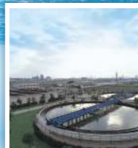
广泛应用于污水处理 Widely used in wastewater treatment
